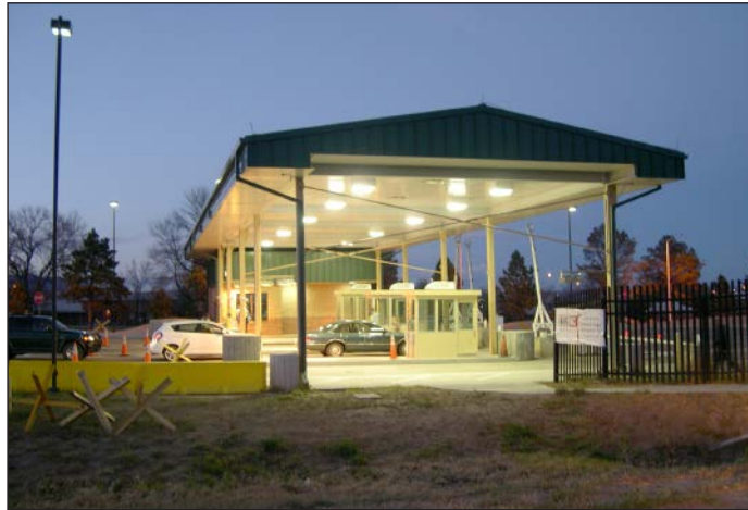
The 9/11 attack caused the Army to relook at its Access Control Points. In response, the Huntsville Center designed new ACPs and supported surveillance and security facilities as well.
