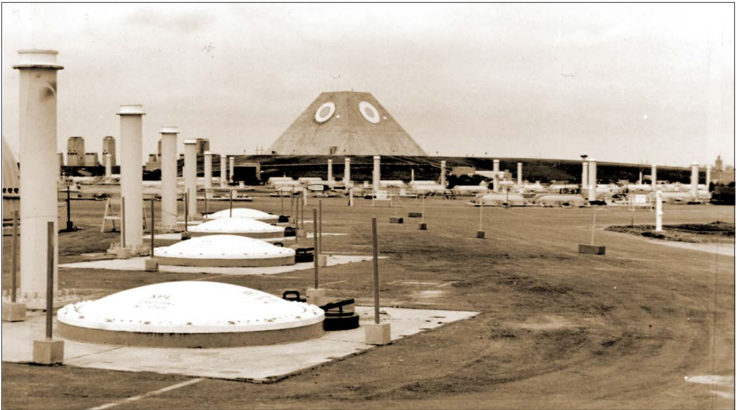
A $468 million construction project, the Stanley R. Mickelson SAFEGUARD Missile Complex near Nekoma, North Dakota, became operational on April 1, 1975 and was the largest single contract let by the U.S. Army Corps of Engineers at the time.
