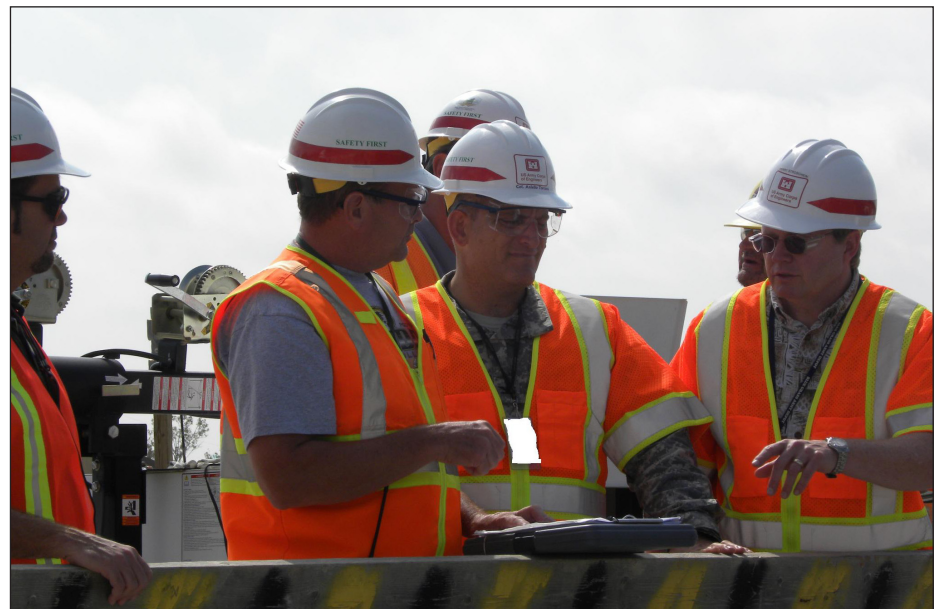
Col. Nello Tortora, Huntsville Center commander, center, visits a construction site at the Bluegrass Chemical Agent-Destruction Pilot Plant in Kentucky.
