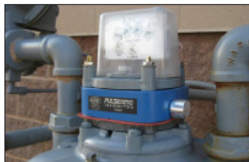
The Utility Monitoring and Control Systems Program designs, procures and installs monitoring and control systems for customers at the Department of Defense and other federal agencies.
