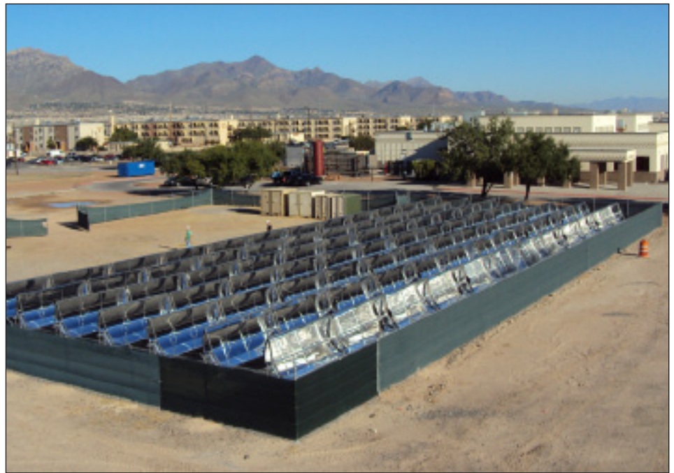
Part of an energy savings performance contract project at Fort Bliss, Texas, a parabolic hot water array was installed to provide preheated domestic hot water.
