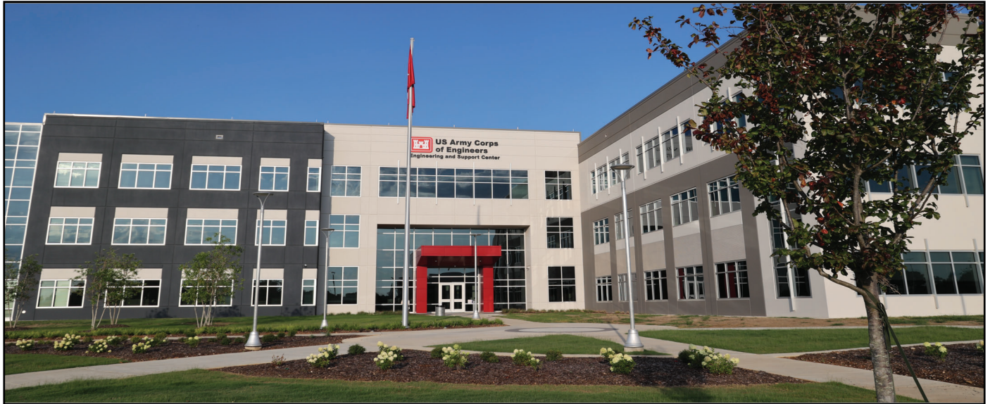
U.S. Army Engineering and Support Center, Huntsville's new building located on Redstone Arsenal, Alabama.
