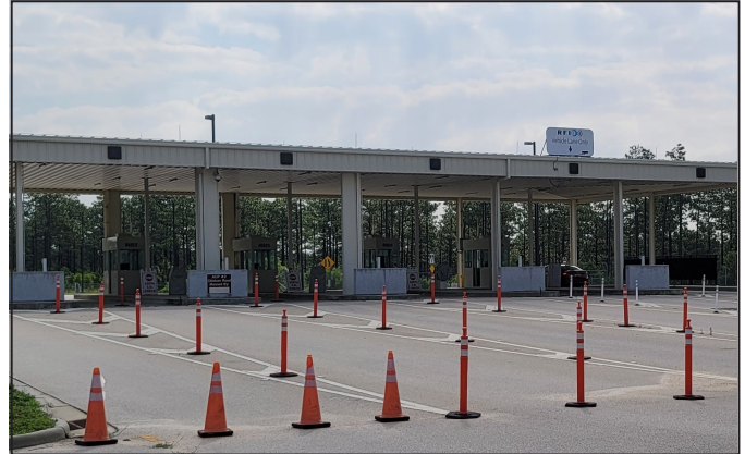
Chicken Road Access Control Point at Fort Bragg, North Carolina, is one of the many Access Control Points to which Huntsville Center maintains and services physical security equipment in accordance with all applicable DOW and agency-specific standards.
