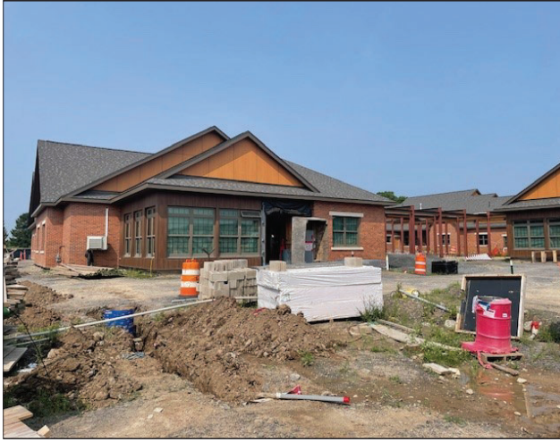
Construction of the Veterans Affairs Community Living Center, Canandaigua, New York.
