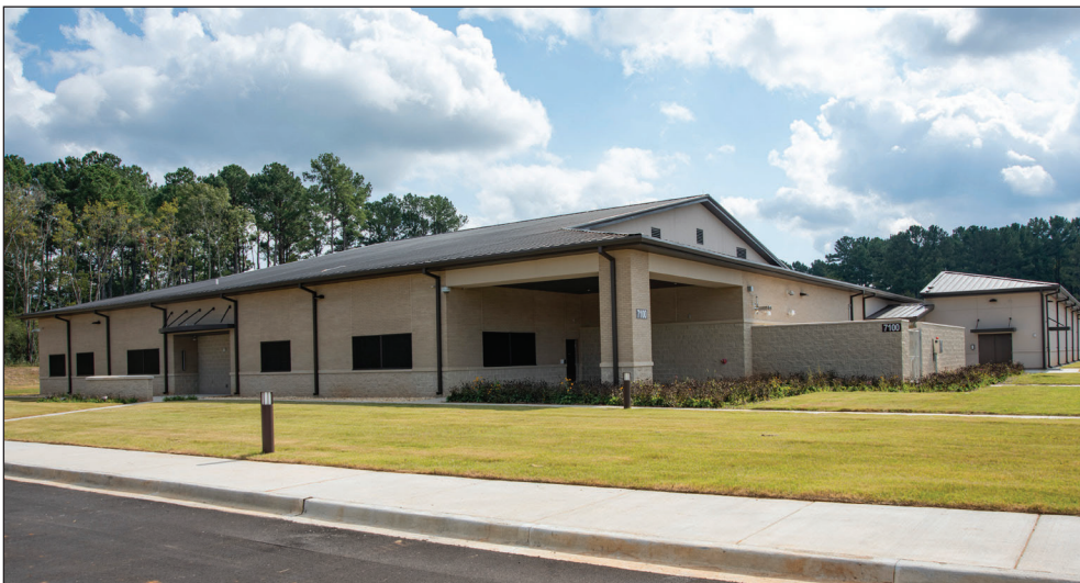
Huntsville Center's FRR Program constructed a new building for the FBI on Redstone Arsenal in Huntsville, Alabama.
