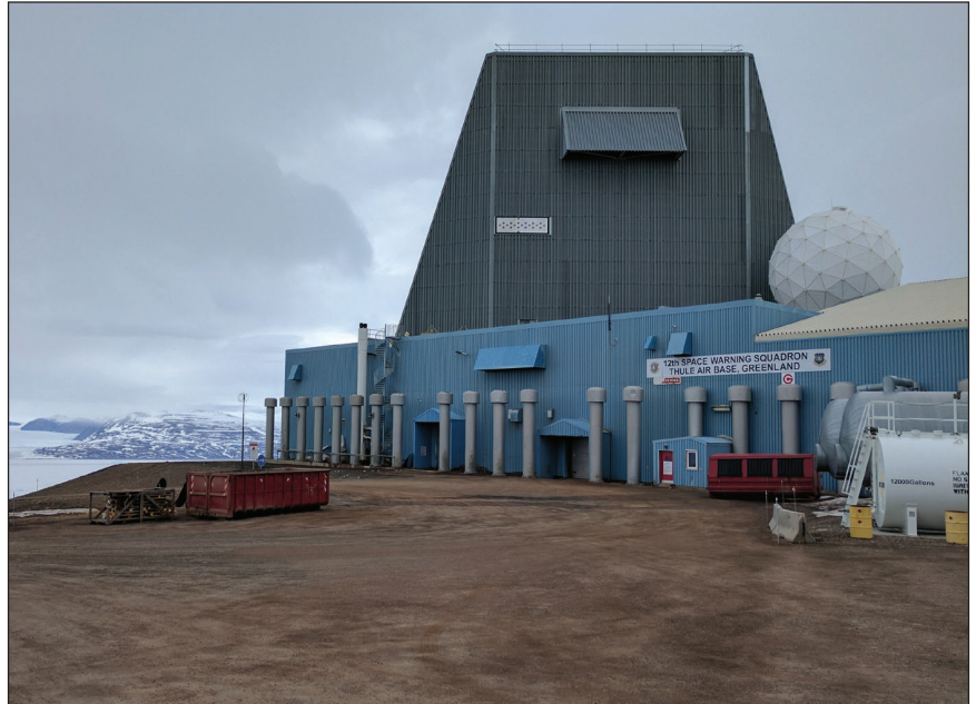
The U.S. Army Corps of Engineers upgraded the High-Altitude Electromagnetic Pulse, HEMP, shield at Thule Air Base, Greenland.
