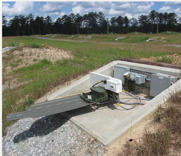
TYPICAL TARGET EMPLACEMENT WITH LOMAH BAR INSTALLED
