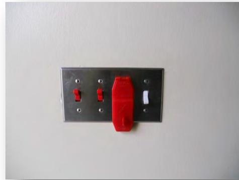
Provide separate switching for the standard and red lighting. Clearly label switches and provide covers over white lights, or similar protective measures, to deter turning on white lights while red lights are in use. Locate switches near points of egress. Provide a means to turn off all exterior white lights including an over-ride for lights controlled by a photocell.
