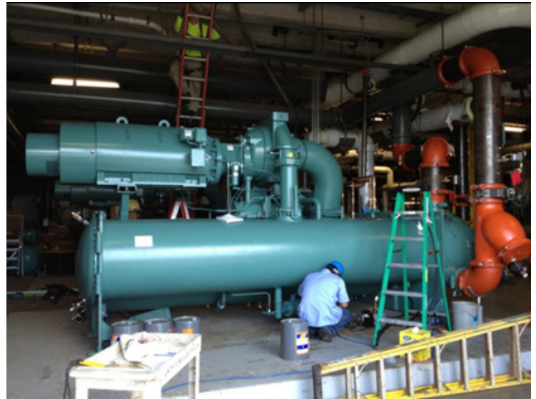
Maintenance is performed on a chiller.
