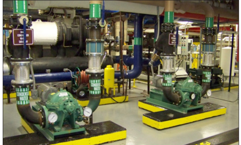
This is an example of pumps found in a hospital mechanical room. The OMEE program maintains the facility and performs preventive maintenance and repairs to these type systems.
