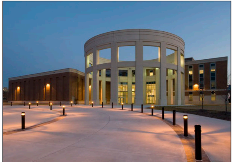
Front entrance to Lincoln Hall at the National Defense University on Fort McNair in Washington, D.C. Huntsville Center's BASEOPS Program supports NDU facility maintenance.
