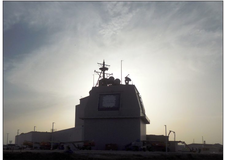
Construction at the Missile Defense Agency Aegis Ashore Missile Defense Complex in Devesulu, Romania, March 2015.
