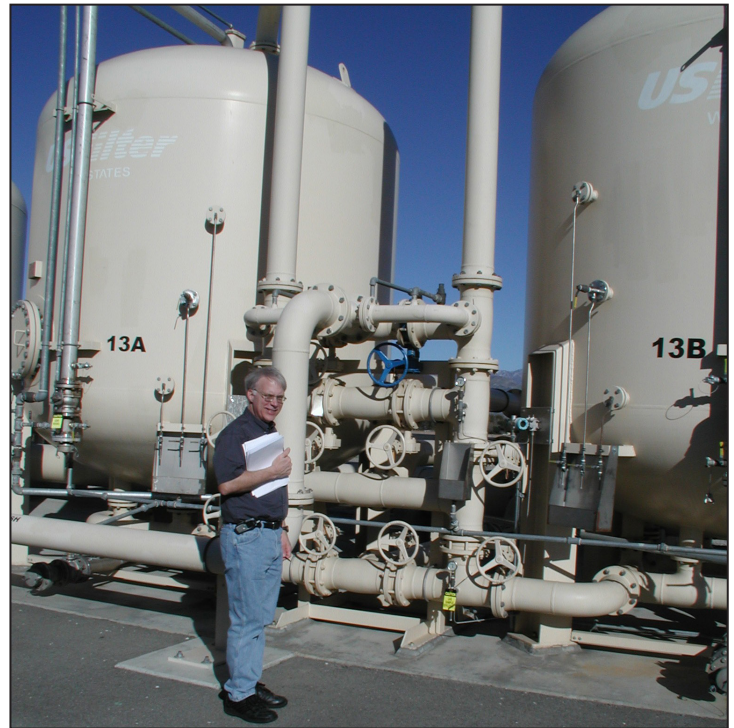
Conducting a site inspection of the treatment plant at the Newmark Ground Water Contamination Superfund Site in San Bernardino, California.
