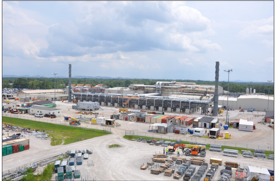
Blue Grass Chemical Agent-Destruction Pilot Plant in Richmond, Kentucky
