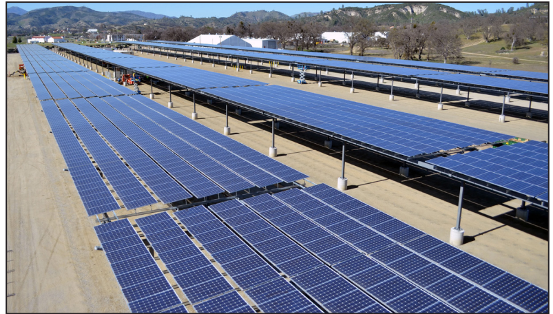
Pictured is an Energy Resilience and Conservation Investment Program solar microgrid project at Fort Hunter Liggett, California, managed by the Sacramento District. A Fiscal Year 2016 ERCIP project added additional rooftop solar panels and a second battery energy storage system.
