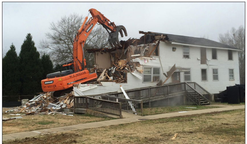
Soldiers Plaza building 2602, a World War II wood building used most recently as an administrative building, is demolished at Fort Benning, Georgia, under the Facilities Reduction Program.
