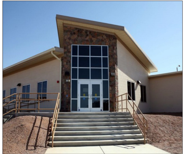
The outpatient clinic renovation at Fort Huachuca, Arizona, was a Medical Repair and Renewal Program project.
