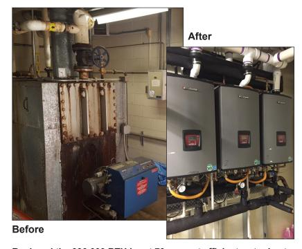
Replaced the 990,000 BTU input 70 percent efficient water heater (left) with 740,000 BTU input 90 percent efficient tank-less water heaters (right) to perform the same water heating requirement.
