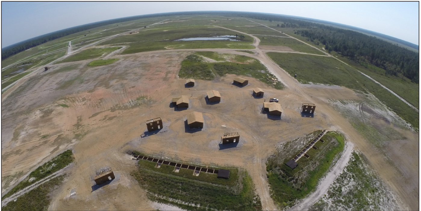
An urban building cluster and trench objective on the Multipurpose Training Range at Fort Stewart, Georgia.
