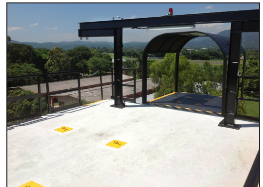
Rappel Tower Retrofits, El Salvador
