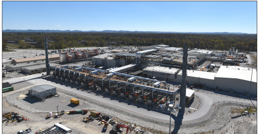
Blue Grass Chemical Agent-Destruction Pilot Plant in Richmond, Kentucky.
