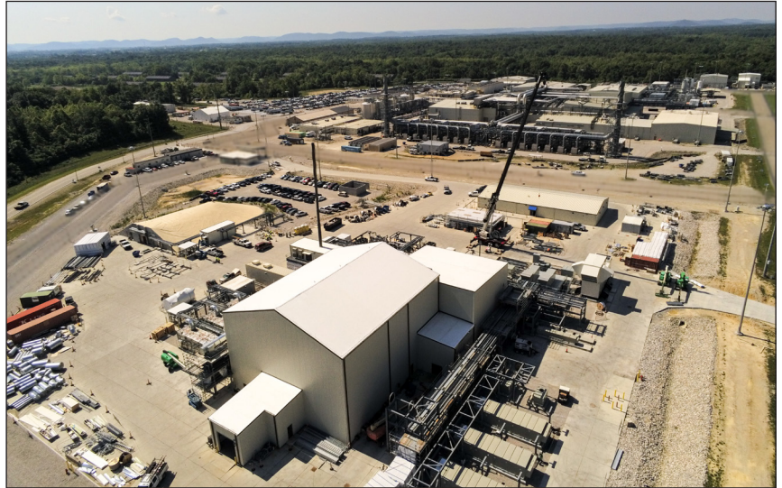
Blue Grass Chemical Agent-Destruction Pilot Plant in Richmond, Kentucky.
