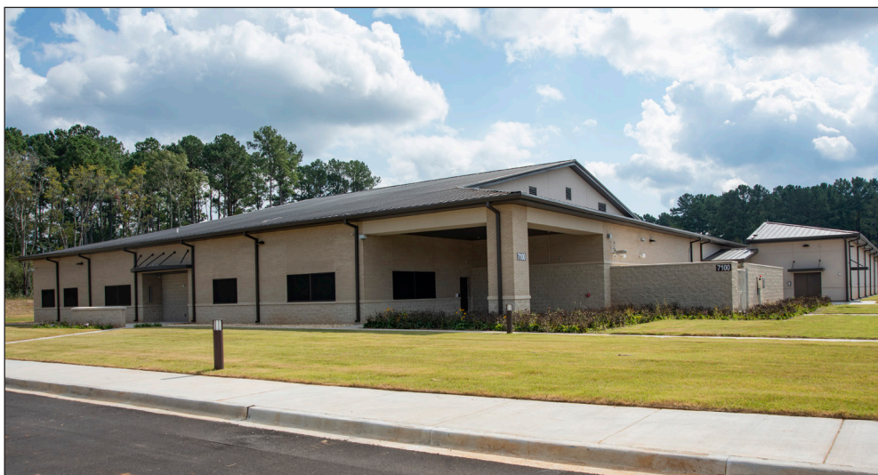
Huntsville Center's FRR Program constructed a new building for the FBI on Redstone Arsenal in Huntsville, Alabama.
