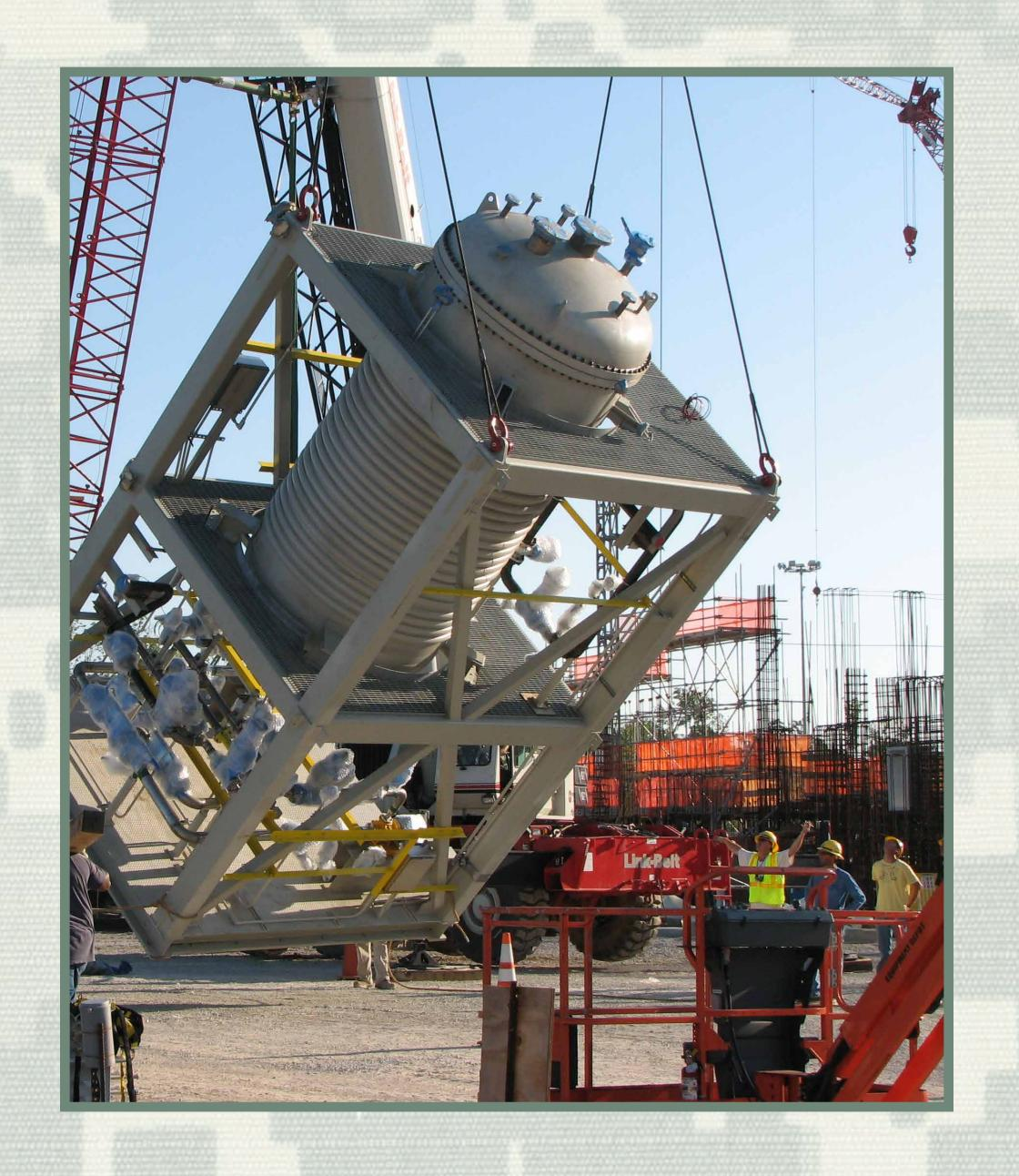
Neutralization followed by supercritical water oxidation was the destruction technology approved by the Department of Defense for the Blue Grass facility. Three energetics neutralization reactors will neutralize chemical agents that have been removed from chemical munitions.
